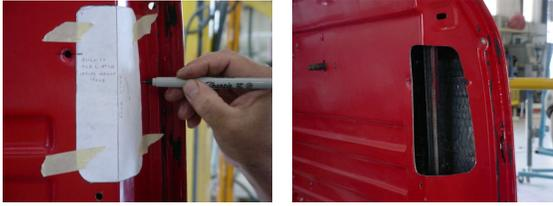
Use the supplied template to mark and cut opening in door. Take the time to align template properly. (Please see blown up image on reverse side of this page).
